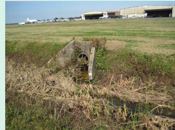
Opening of storm water culvert
